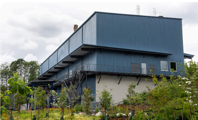
Corix biomass plant
