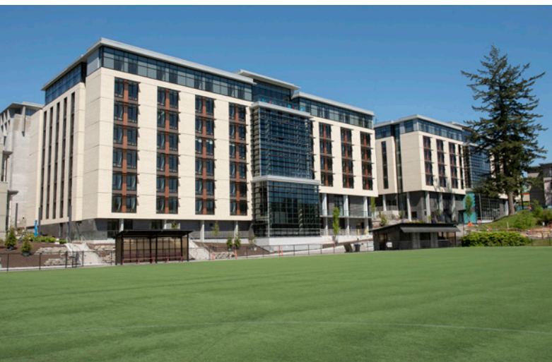
Phase 1 of our new student residence buildings
